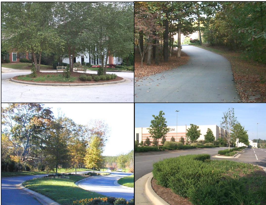
Figure 2.18 Example of Reducing Impervious Cover (clockwise from upper left): (a) Cul-de-sac with Landscaped Island; (b) Narrower Residential Street; (c) “Green” Parking Lot with Landscaped Islands; and (d) Landscape Median in Roadway.
