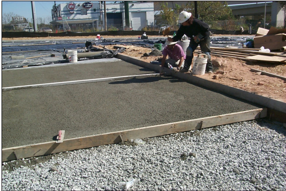
Figure 25.2 Porous Concrete System Installation
