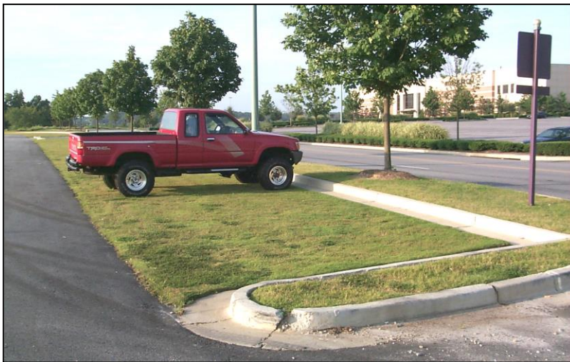
Figure 2.22 Grass Paver Surface Used for Parking
